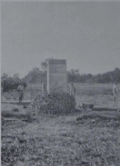
AS LEFT AFTER WORK.
